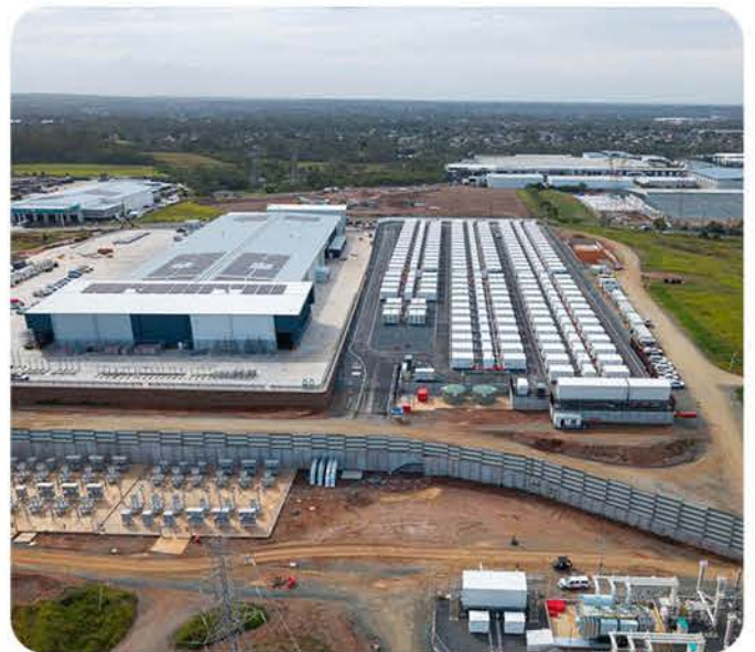
Supernode project in Brisbane's northern suburbs.
